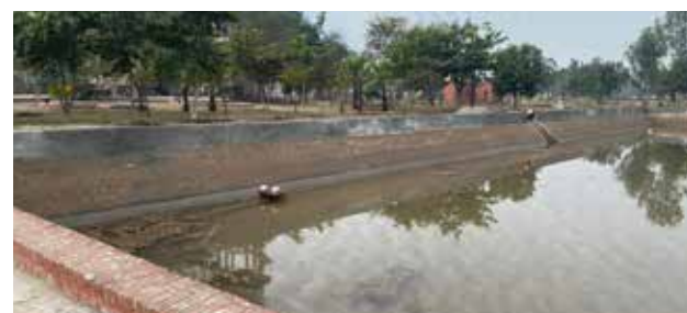
Renovation of water works
